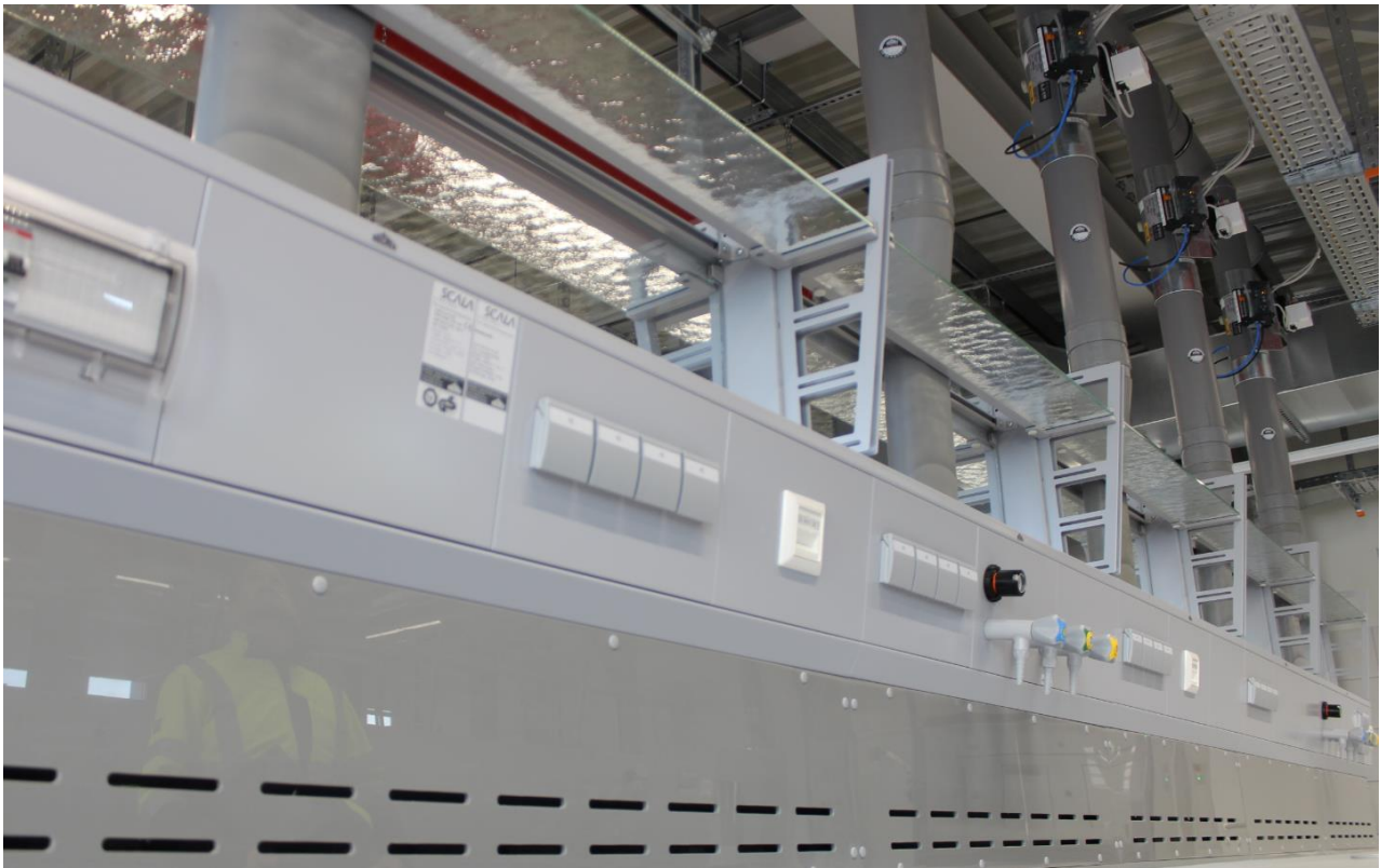
Figure 4: Test laboratory in accordance with the most modern standards: All workstations are also equipped with fume cupboards and exhaust slots, which continuously extract air from the laboratory benches. Zeller+Gmelin's new QC laboratory is also equipped with various connections for technical gases, so that an extension of analytical determinations can be realised at any time.
