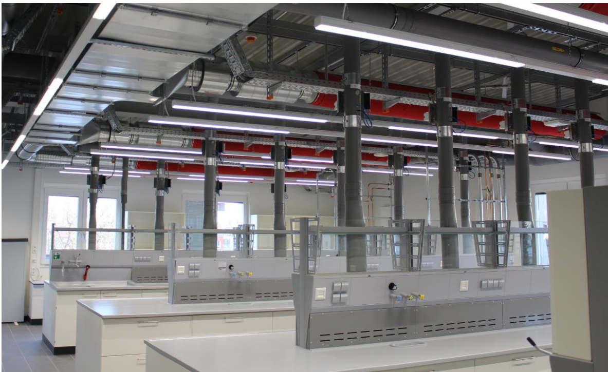
Figure 2-3: Air supply through textile air distribution systems: The new premises are equipped with a generous number of fume cupboards so that work with chemicals that are hazardous to health or have a strong smell can be carried out under optimum conditions.
